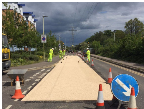
High friction/anti-skid road surface being applied
