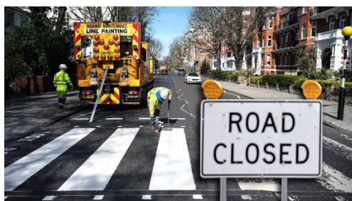
Lining and road markings
